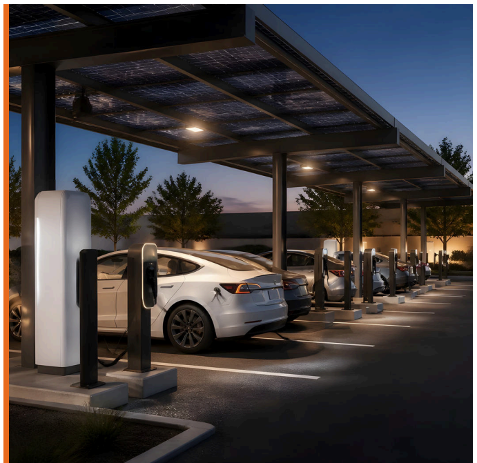
EV: solar carport with AC and DC fast chargers
