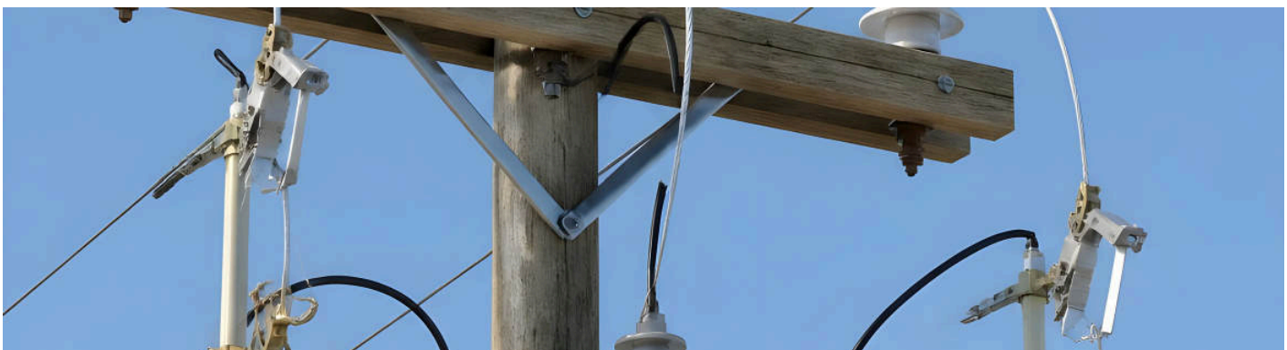
Application: pole-top distribution transformer with hot-line clamps, cutouts and arresters.
