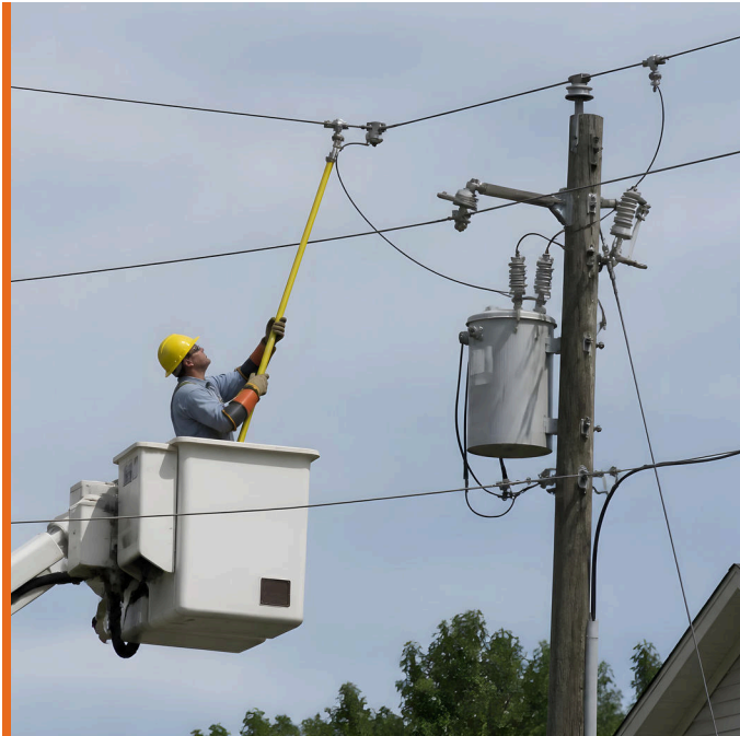
Overhead tap: a lineman sets a hot-line clamp on the energized primary with a clamp stick from an insulated bucket
