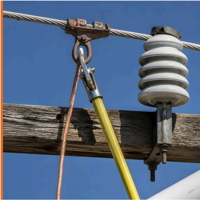
Hot-line clamp: main groove on the primary (or a stirrup bail on 336 ACSR and larger), tap jumper in the eyebolt, set with a clamp stick
